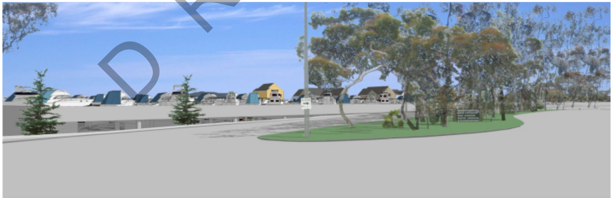
Figure 4D: Dry Boat Storage Deck Driving West on Dana Point Harbor Drive at the Puerto Place intersection
